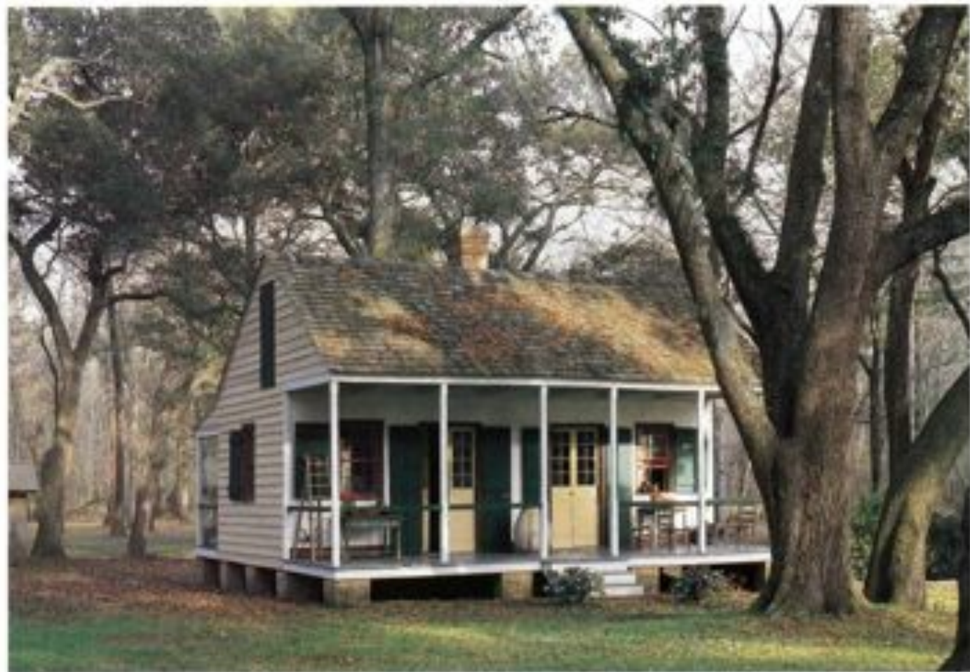
above: A glassed-in back porch looks off to a stand of ancient live oaks on Smith's nine-acre property. above: The little house, built circa 1838, was probably a Creole plantation family's weekend house in Saint Martinville, seat of Saint Martin Parish. The French floor plan sets a salon and bedroom side by side. Both rooms open directly onto the deep front porch through glazed double doors and are served by the central chimney.
